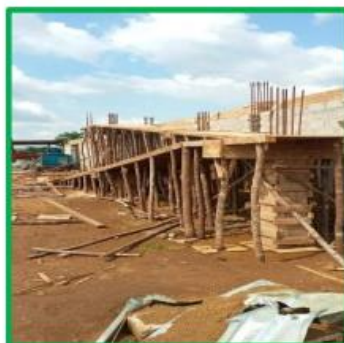
View of formwork for ramp
