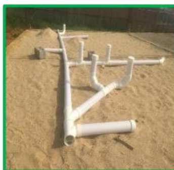
View of rough plumbing for foundation
