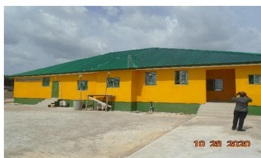
Rear View of the Building
