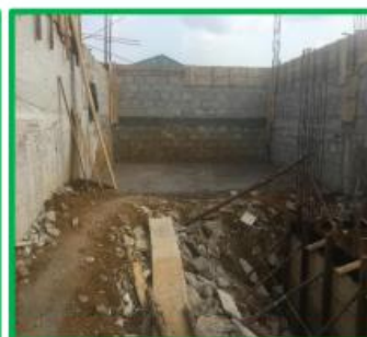
View of basement being prepared for stair
