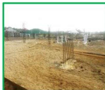
View of foundation with stair starter
