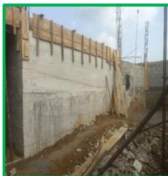
View of formwork for basement beam
