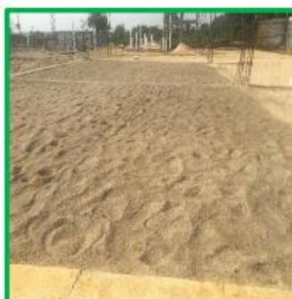
View of backfill in foundation
