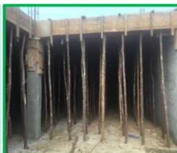
View of round poles as support for basement formwork
