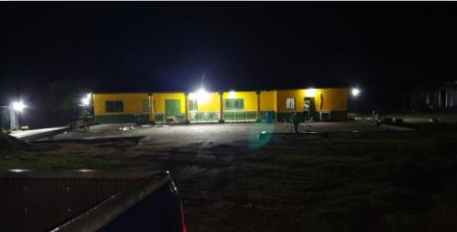
Night view of the Lab – powered by Solar Panels
