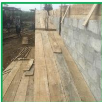
View of formwork for access ramp
